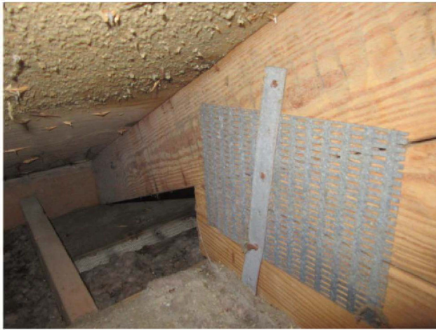
Roof to Wall Attachment - Clips
