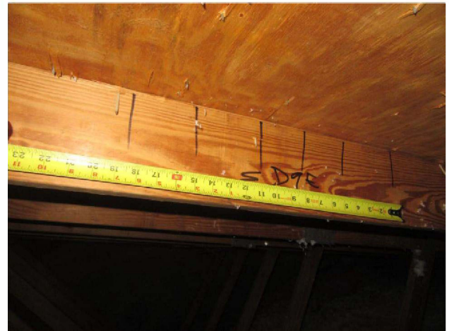
Roof Deck Nail Spacing - Field
