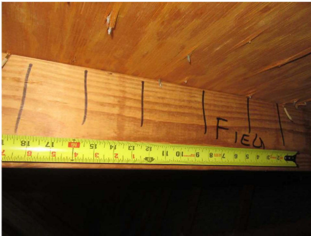
Roof Deck Nail Spacing - Edge
